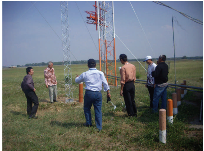
Installation of the Primary sensor group tower
