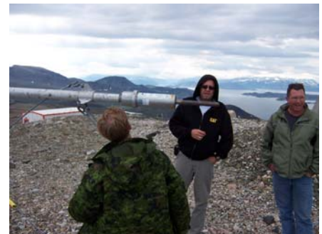
The old wind monitor is removed to make way for the new
