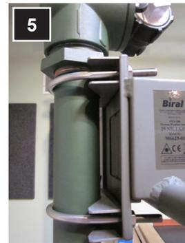
5. Mount the **Visibility Sensor** to the top tower section, just below the junction box.
