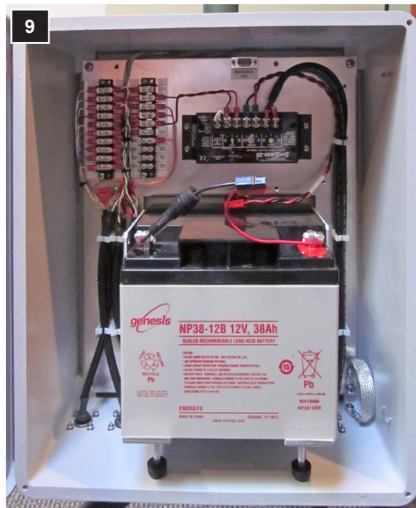
8. Mount the **Power Supply (Battery Box)** to the lower tower using the clamps on the rear of the enclosure as shown.
